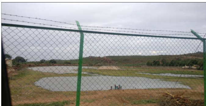
Shirur Big Water Tank
